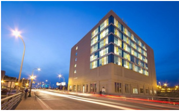
Mark's renovated building in downtown Syracuse, NY
